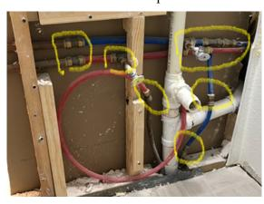
During the demo I found at least 20 shark bite fittings in areas where there should have not been any. Just in this small area there were 11 shark bite fittings. Each one with a chance of failure at some point. I'm now having a plumber put in all new pipe in my kitchen and utility room.
